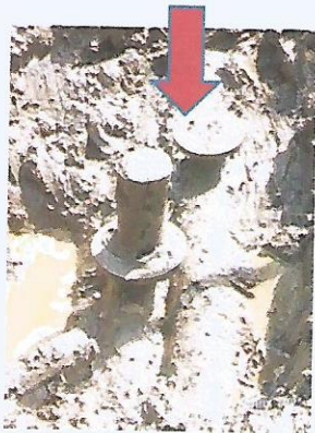
Pic1: Showing 2nos 3" valves installed on the pipeline
